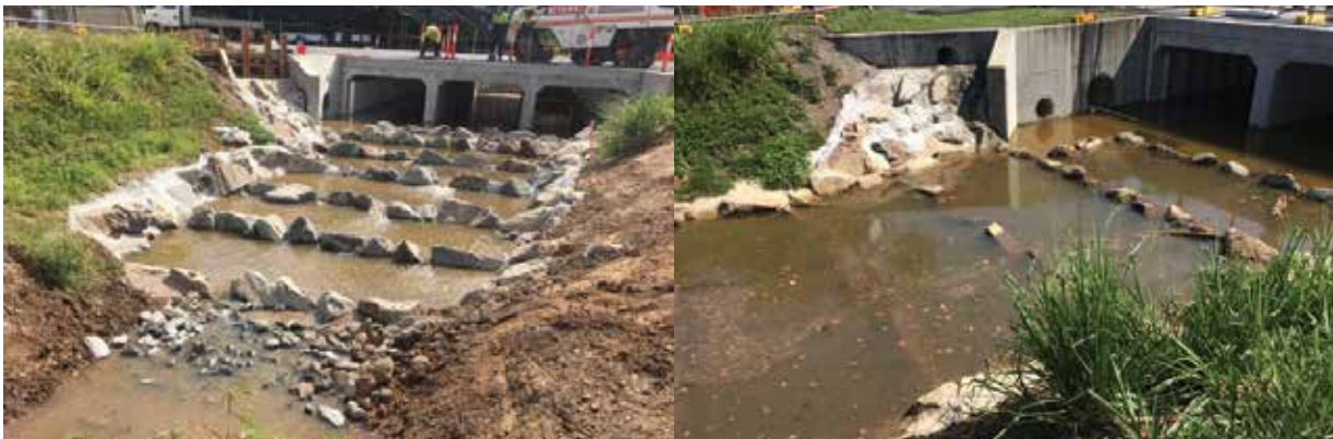
Fishway Ladder installation on Swallow Street
