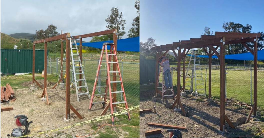
Figure 8&9. 4"x6" Beam and Rafter Framing
