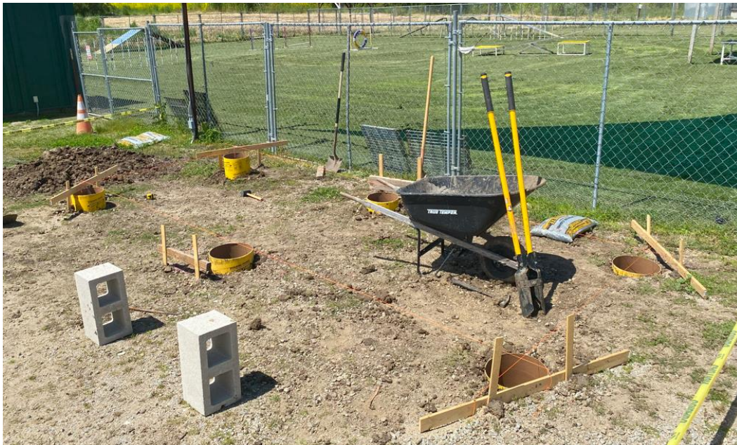
Figure 4. Formwork Set
