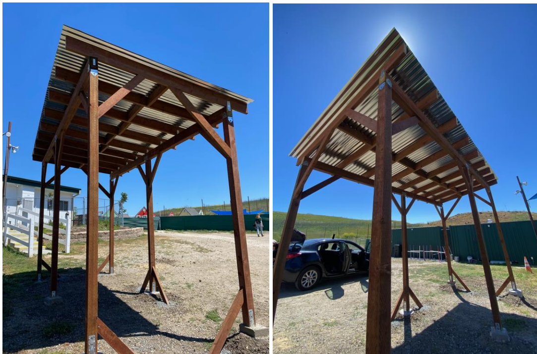
Figure 1&2. Completed Lean to Shade Structure
