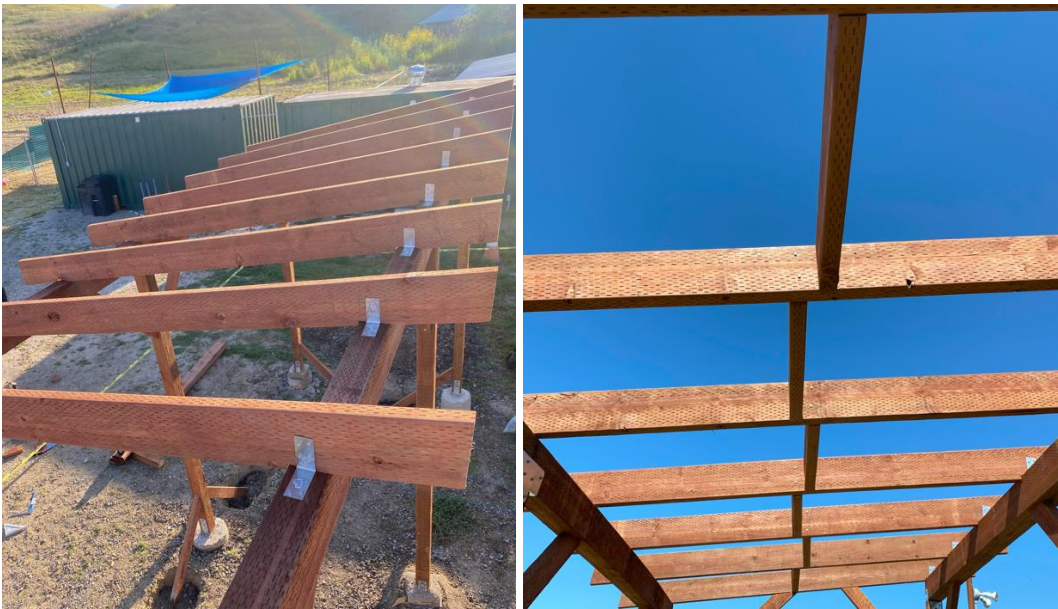
Figure 10&11. 2"x6" Rafters (Left) and Blocking (Right)
