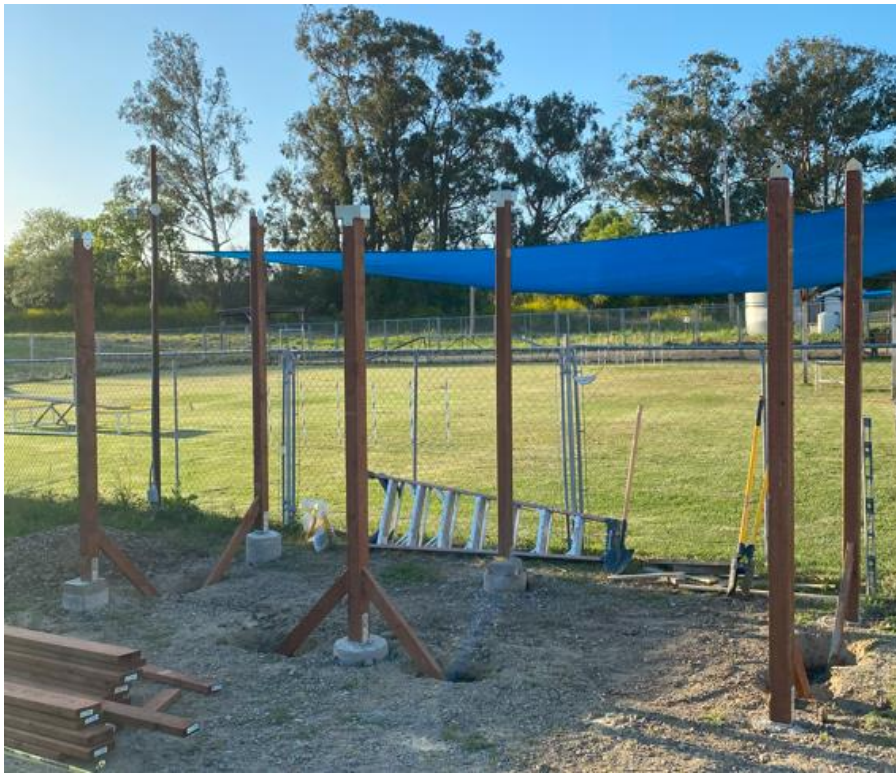
Figure 8. 4"x4" Posts and Embedded Cross Braces Set
